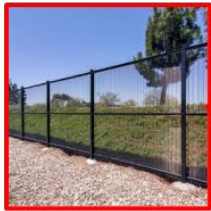
8' TALL SECURITY FENCE W/ FIRE ALARM INTEGRATED GATES
