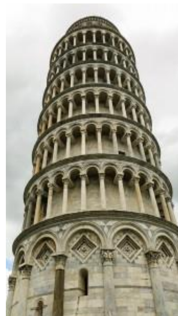
Leaning Tower of Pisa
